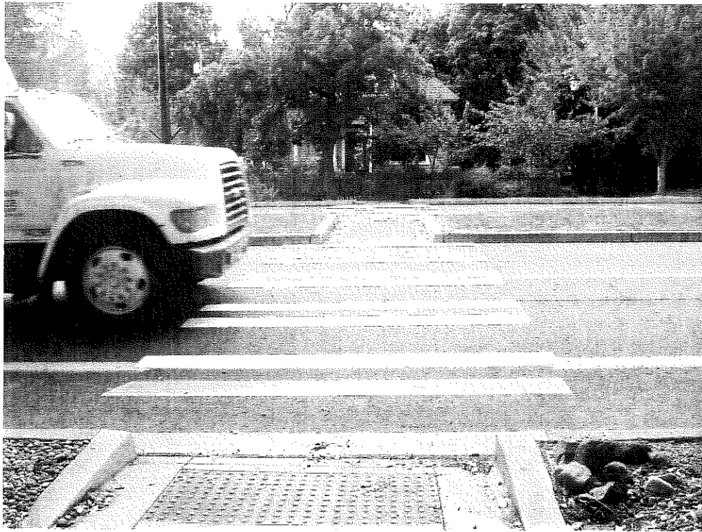
Existing crosswalk at Harrison Street
